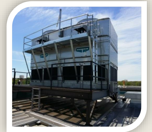
Cooling Tower Replacements
